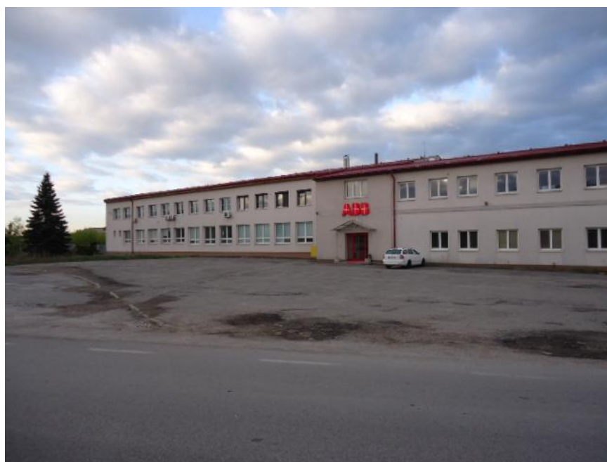
Fig. 3 ABB office building.
