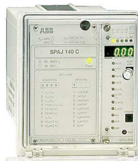
Figure 3 Overcurrent and earth-fault relay SPAJ 140 C [5]
